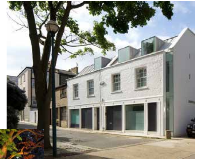
Mews type facade with mix of large openings to Ground floor and sash windows to 1st floor
